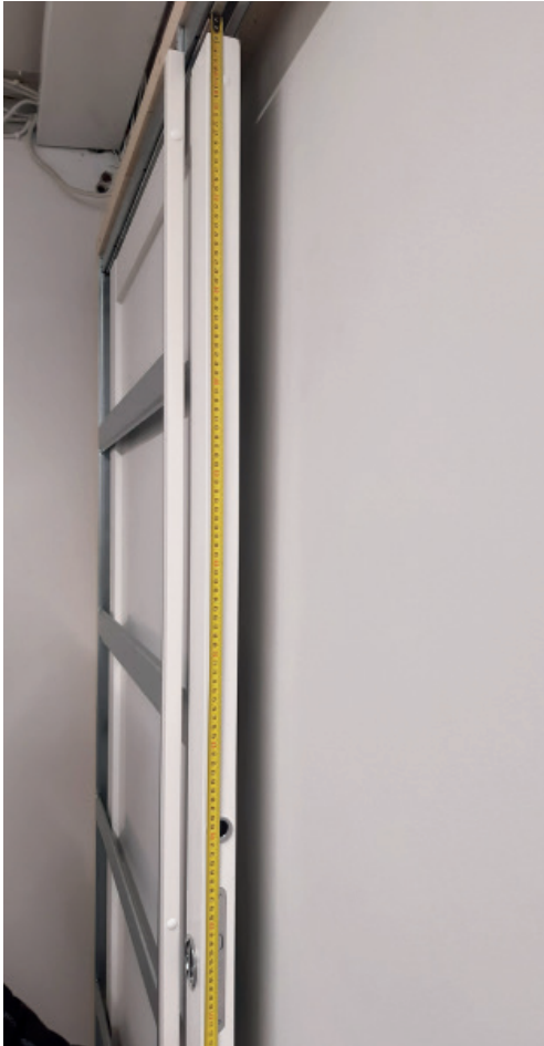
1A. When the door is adjusted, take a measure from the top rail to the top edge of the locks tongue.
