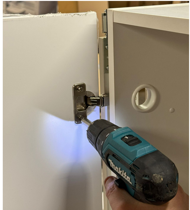
23. Finally, attach the doors to the hinges.
