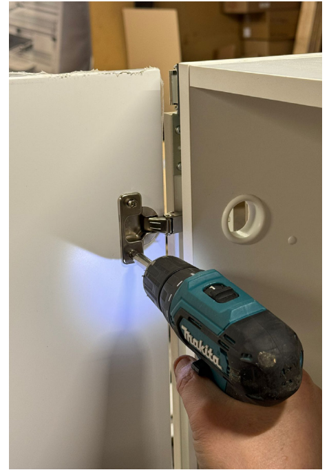
24. Finally, attach the doors to the hinges.
