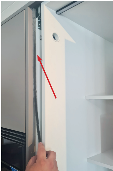
23. Pull out the hinges plate to the outermost position and attach the brush seal along the front edge.
